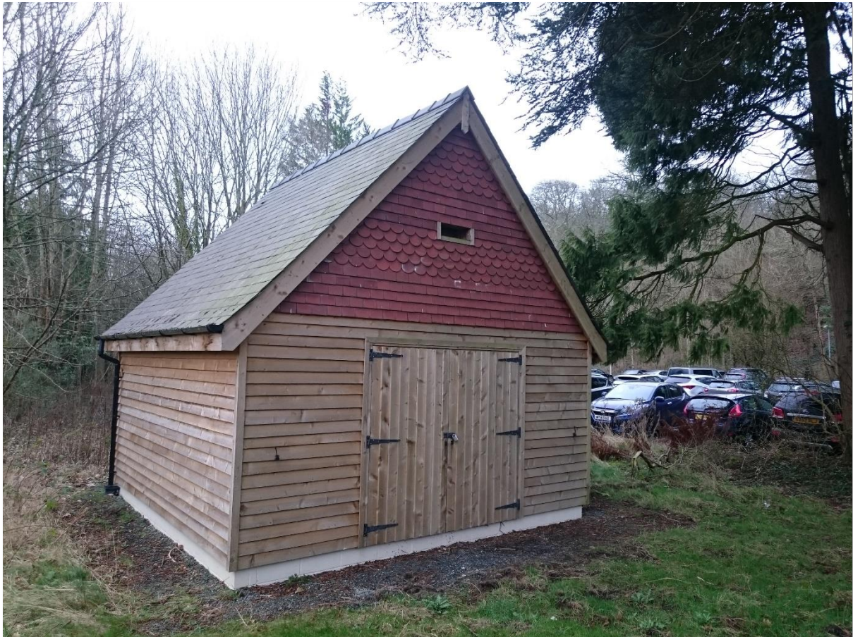
Figure 2.1. New bat roost incorporated above a storage shed at the former Southfields site, Llandrindod Wells, 2017.
